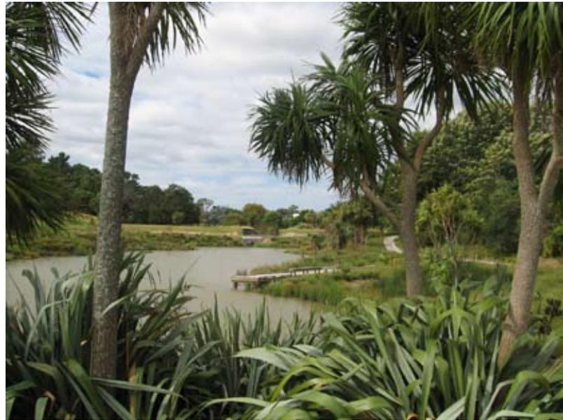
Re-contouring provided for a planted buffer and safety shelves to the pond while accommodating the required storage capacity.
