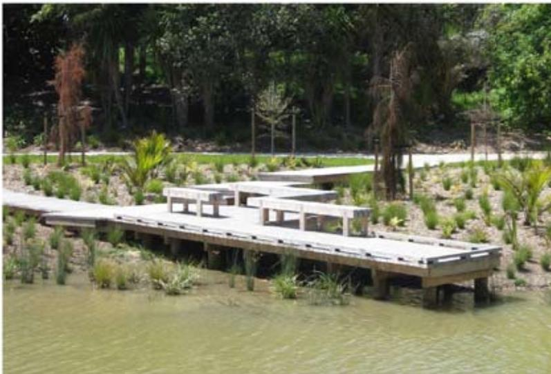
A boardwalk platform provides proximity to the wetland. *Macrocarpa* was used in place of treated pine or sustainable tropical hardwoods (in limited supply). Similar to other aspects of the project the boardwalk platform mirrored NSCC park standards for decks, but were a bespoke design. The vegeta-
